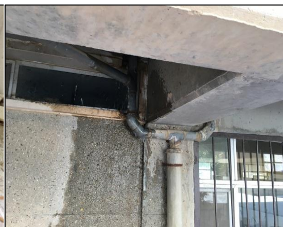
Figure 4: the old sewage pipes (2) inches
